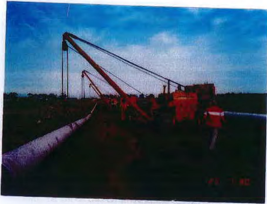
Snaking in a 500 mm diameter pipe near the Mossgas Refinery
