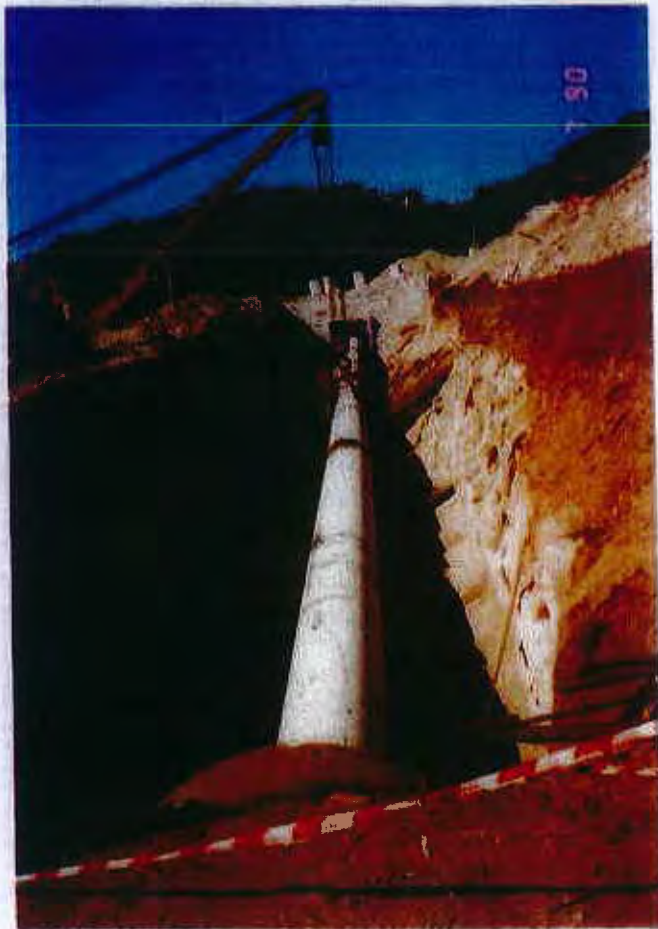
800 mm diameter pipe crossing a provincial road
