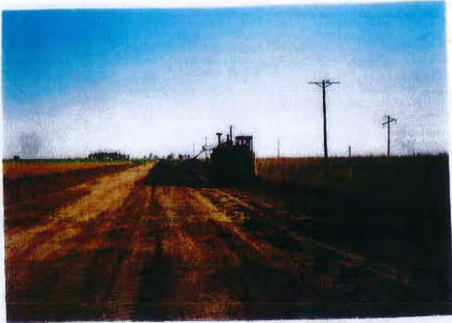
Trencor Jetco. Trencher in operation.
