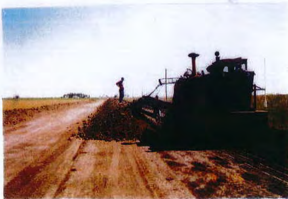
Close up of Trencor Jetco in operation.
