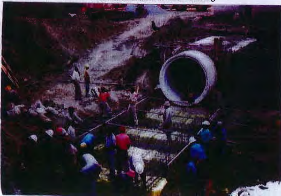
Encasement of sewer pipe at a river crossing
