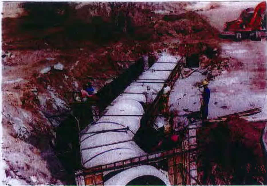
Bend encasement at river crossing
