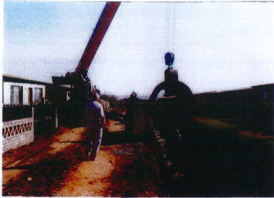
Boksburg - Brakpan April 1987 to July 1988 Laying a 1350mm diam sewer in a built up area
