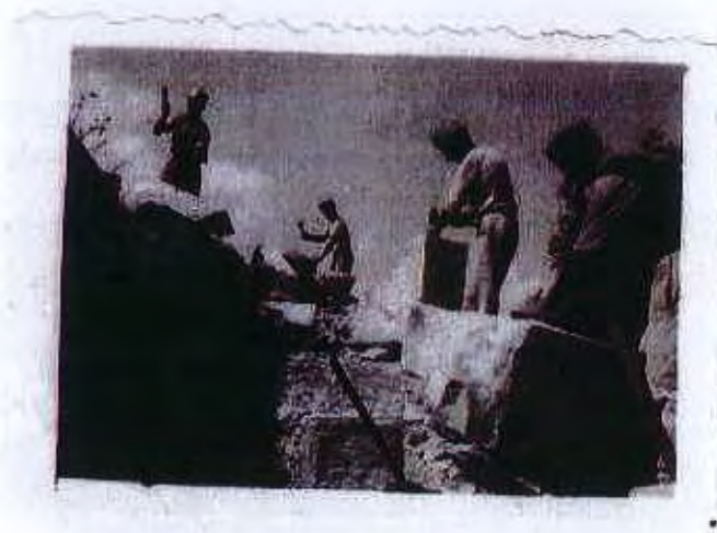
Stone masons shaping stones for the river Trigno Bridge - Italy
