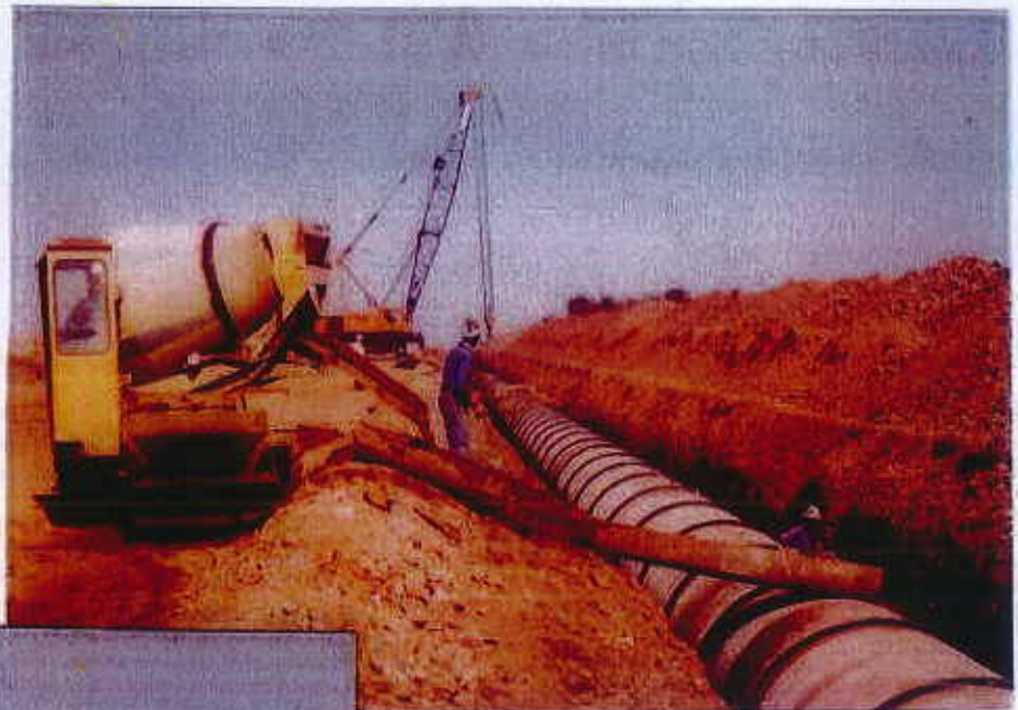
Placing soil crete at base of pipe
